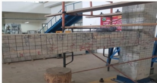
Fig. 5. Crack Pattern of STR-1
